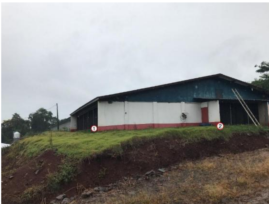
Figura 48: Sistema de resfriamento – Pad cooling . (1) Painel evaporativo pad cooling – face 1. (2) Painel evaporativo pad cooling – face 2.
