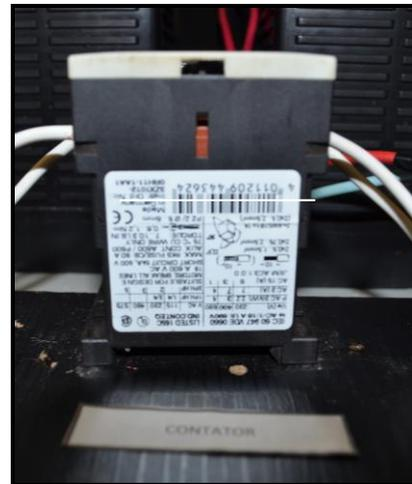
**Figura 34** – Contator SIEMENS – Vista lateral.
